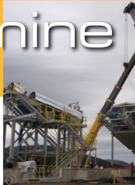
A Grove RT765E rough-terrain crane helps construct a balloon structure for an ore storage silo at a Fermont mining site in Quebec, Canada.
