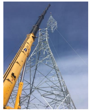
350 T hydraulic crane – Electrical tower installation – Hydroelectric powerplant La Romaine-4 – Near Havre-St-Pierre March 2019 (Picture : Ian Corbin, crane operator)
