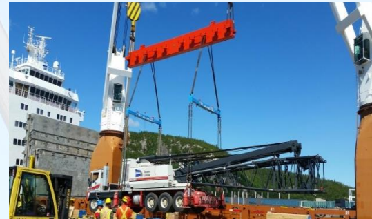
Loading of the 300 ton Link-Belt truck mounted at the Port of Baie-Comeau
